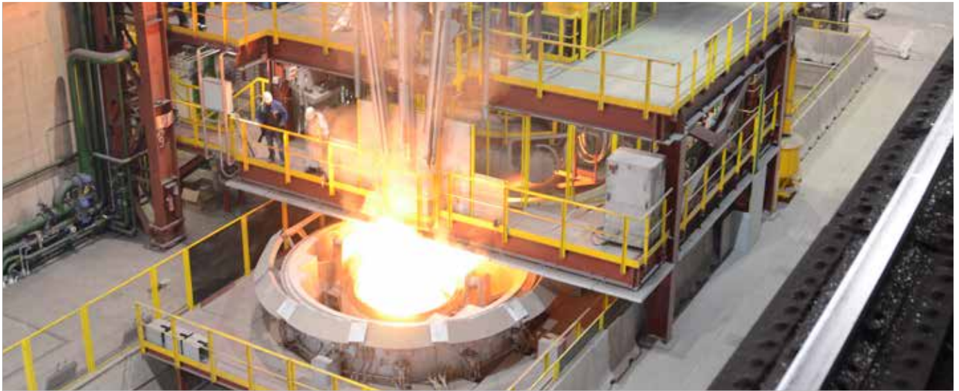
Efficient and reliable solutions for VOD and VD-OB plants
