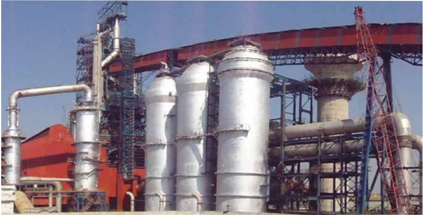
JSPL Angul Blast Furnace No.1
