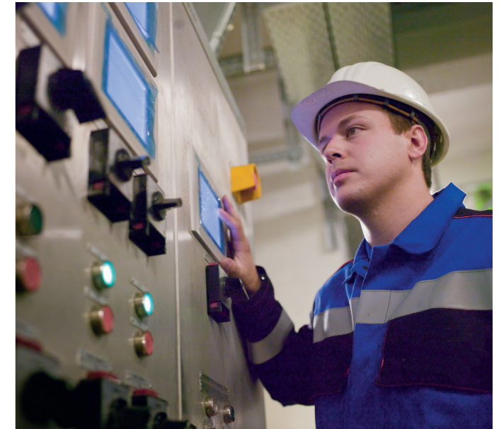
Inspection performed by a Primetals Technologies electrical engineer
